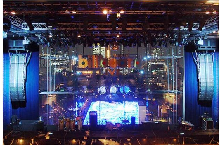
controlled low-end distribution across all three floors. Along with the VTX Series line array speakers and subs, Hibino deployed VTX-F12 loudspeakers as outside fills to provide even coverage on the far sides of the stage. Utilizing the same D2 Dual Driver technology as the VTX Series, the VTX-F12 blends seamlessly with the main speakers while providing wider horizontal coverage. In order to provide crystal-clear monitoring on stage, Hibino deployed VTX-M20 speakers as floor monitors.
